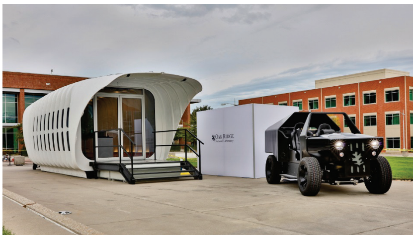
Bidirectional wireless charging technology enabled energy to flow between this novel printed vehicle and building as part of the Additive Manufacturing Integrated Energy demonstration project.
