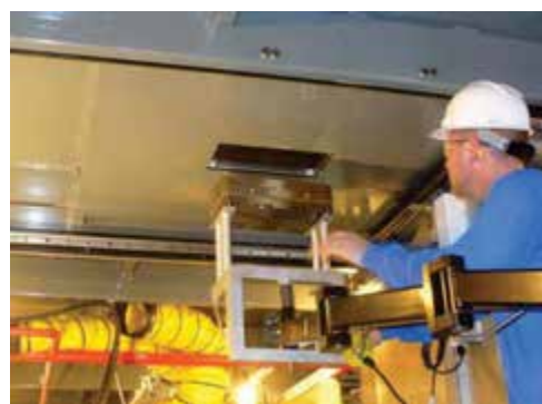
Spin pack installation on the melt spinning semi-production line.
