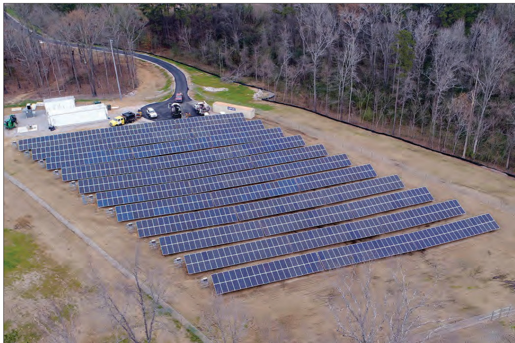
The microgrid includes 11 rows of solar panels with more than 1,200 modules that convert light from the sun into energy. Solar panels can supply power to both the neighborhood and existing electric grid. Photo courtesy: Southern Company
