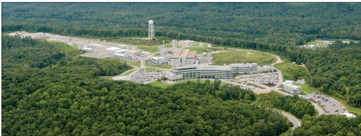
The Spallation Neutron Source. Image: Jason Richards, ORNL
