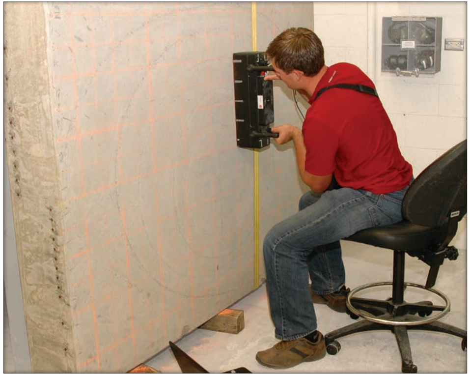
University of Minnesota researcher Kyle Hoegh positions an ultrasonic linear array on a test wall section. The device uses sound waves to examine the internal condition of concrete structures. Image credit: Dwight Clayton, ORNL
