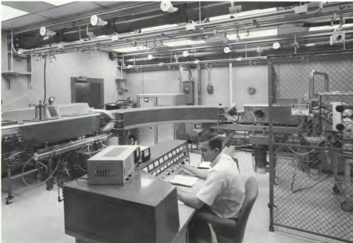
Curt Bemis at the controls of TRL's electromagnetic isotope separator.
