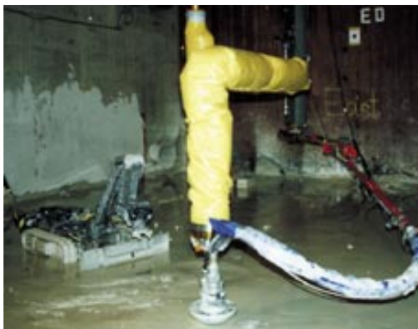
The Houdini (left) and MLDUA (center) are among the components of the RTCS that work together to effectively clean a tank's interior. Image provided by the Gunite Tanks Remediation Project.
