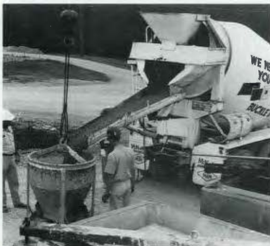
The concrete box holding radioactive waste is filled with cement to further immobilize the material.
