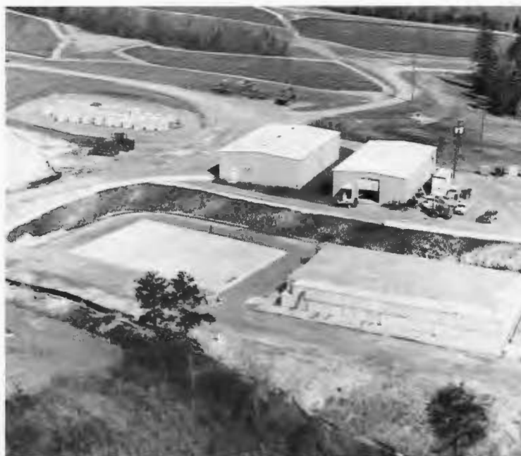
The tumulus facility comprises stacks of waste boxes on a concrete pad. The boxes are then covered with more concrete, plastic liners, and soil to keep water away. At top is Solid Waste Storage Area Number 6.
