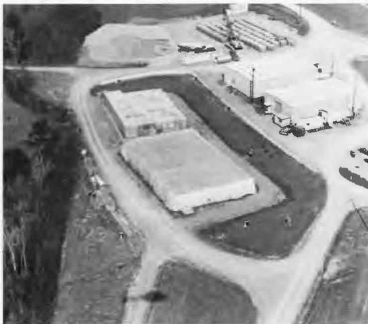
The first pad of the tumulus facility is full, and its waste boxes are covered with a plastic sheet. The second pad is rapidly filling up with concrete boxes containing low-level radioactive waste from ORNL.
