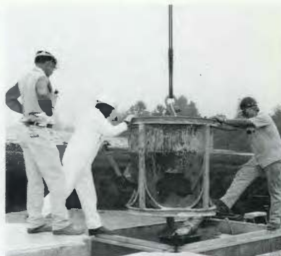
The concrete box holding radioactive waste is filled with cement to further immobilize the material.
