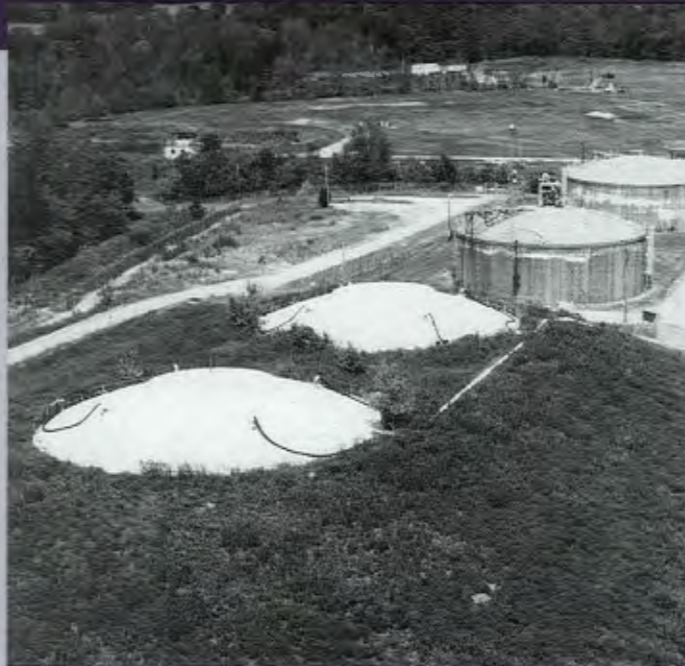
The storage silos at DOE's Fernald Feed Materials Production Center were built in 1951 to temporarily store radium-rich uranium ore. Discovery of the health hazards associated with radium prolonged this stay by several decades.
