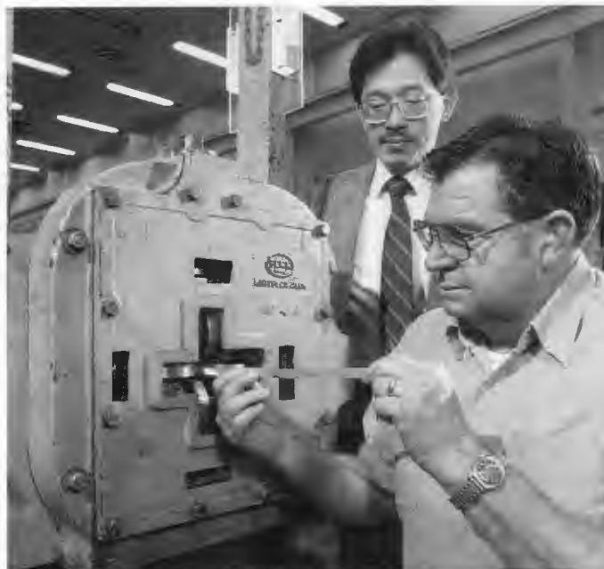
Huey S. Hsu, former ORNL researcher and a consultant to American Superconductor, watches Charlie Dunn, a technician in the Metals and Ceramics Division, extract a thin ribbon of lead-doped bismuth superconducting material. This wire is produced in the laboratory apparatus by rolling and compressing a tube containing powder. Short superconducting wires have been made at ORNL, and their electrical performance has surpassed DOE goals.
