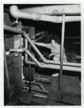
Glenn Wilson (formerly of ESD, now at the University of Tennessee) checks the water flow in the subsurface weir.
