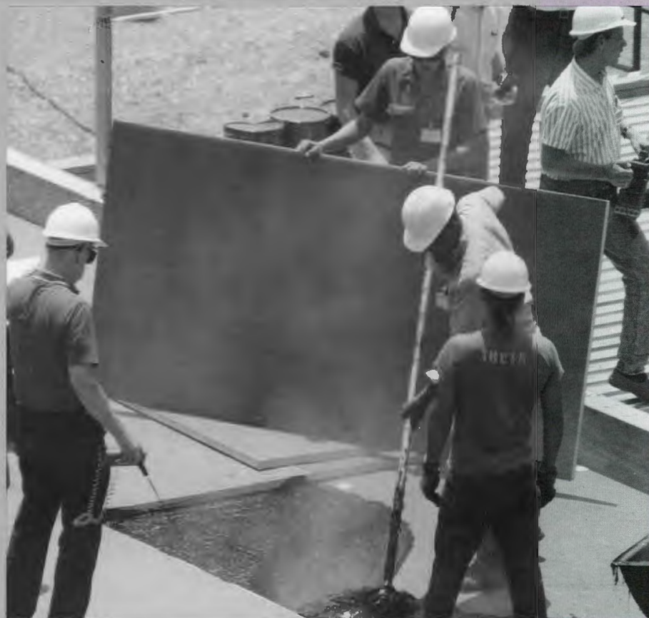
Roofers spread hot asphalt before putting into place a test roof panel containing hydrochlorofluorocarbon (HCFC) insulating gas at ORNL's new Envelope Systems Research Apparatus. Researchers will compare the encapsulation effect of asphalt with that of a laminated membrane over the long-term performance of these foam insulation boards. The HCFC panels pose less of a threat to the stratospheric ozone layer than do CFC panels.
