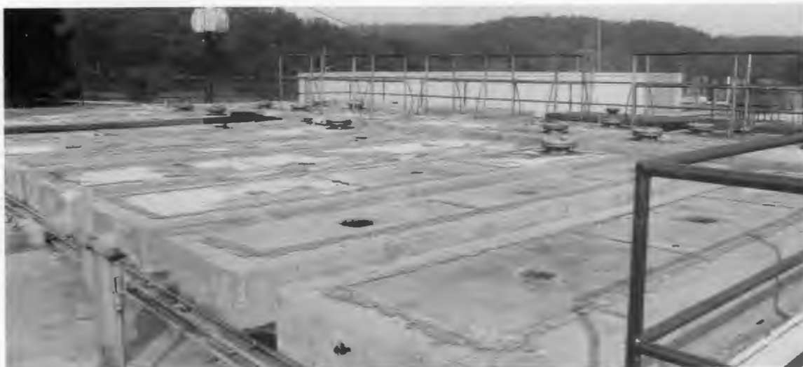
Caps are placed on leaking plugs in the roof of the filter house for ORNL's Graphite Reactor as part of ORNL's effort to upgrade facilities for health and environmental protection.
