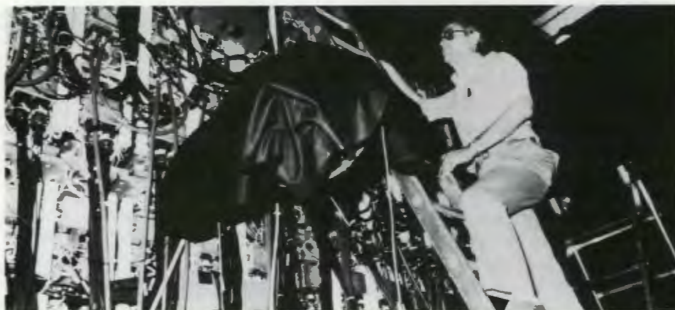
ORNL technician Dick Cumby climbs the ladder to replace one of the 720 phototubes in the ORNL-designed, 60-ton Wall Calorimeter (seen from rear) at the CERN accelerator complex in Geneva, Switzerland.
