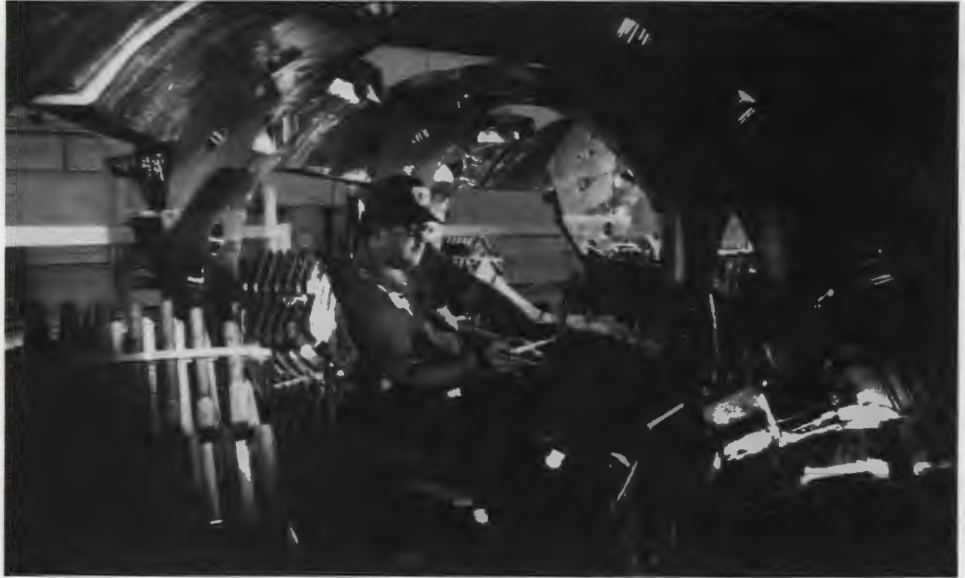
A. D. Cofer of Y-12 Maintenance works inside the ATF structural shell. The lower segments of the ATF helical coils are visible. The upper segments will be reassembled after installation of the ATF vacuum vessel.
