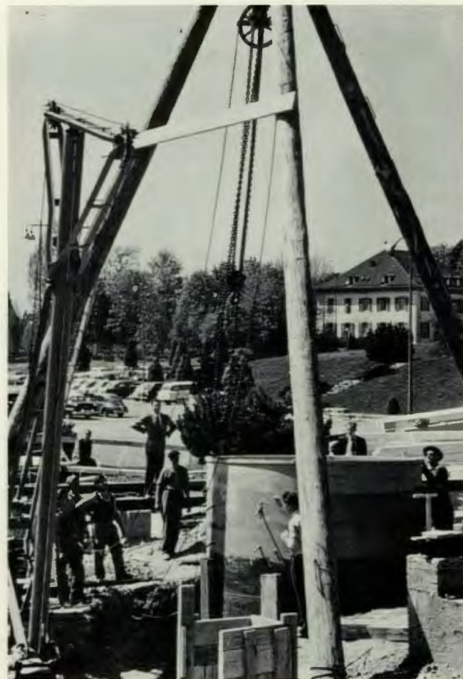
Lowering of the tank into the ground. The building was constructed around it while the reactor was being installed.
