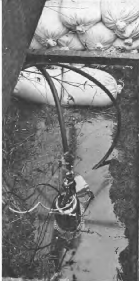
The flow from this storm drain south of a manhole where strontium-90 contamination was detected is blocked by sandbags added by ORNL personnel. Two pumps (one for high flow, one for low flow) pump the water over a wall to the compartment, the contents of which is pumped to the 3524 basin (feed basin for ORNL's Building 3544), where it is treated. The source of the contamination, which occurred in November 1985, was an exposed storm drain pipe at a construction site that broke during a heavy rain.
