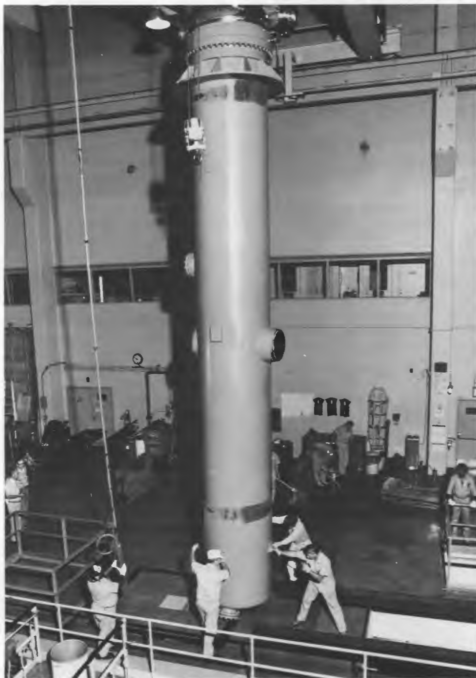
Primary heat exchangers are replaced at the High Flux Isotope Reactor as part of a continuous maintenance program to improve performance and safety. One heat exchanger was replaced in August; the other, in November 1985. This labor-intensive project involved detailed planning and the coordination of various divisions at ORNL.
