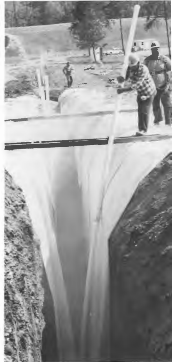
Construction of a French drain at ORNL to demonstrate collection and diversion of groundwater to prevent its contact with down-gradient buried radioactive waste.
