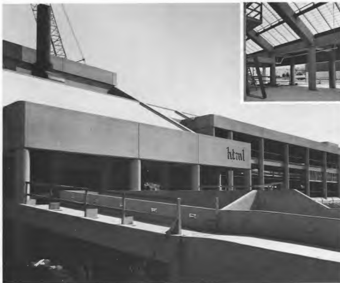
ORNL's $19-million High Temperature Materials Laboratory, which could be ready for partial occupancy in September, makes extensive use of skylights for interior lighting (inset).
