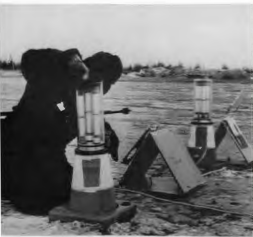
U.S. Air Force employee installs a tritium light developed at ORNL on an Alaskan airstrip.
