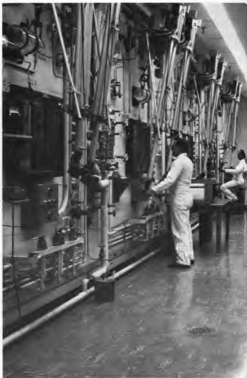
For two decades ORNL was an isotope production center. Here, clockwise, Bob Byrum, W. G. Tatum, and Tom Rice use master-slave manipulators in hot cells for preparing isotopes for customer use.
