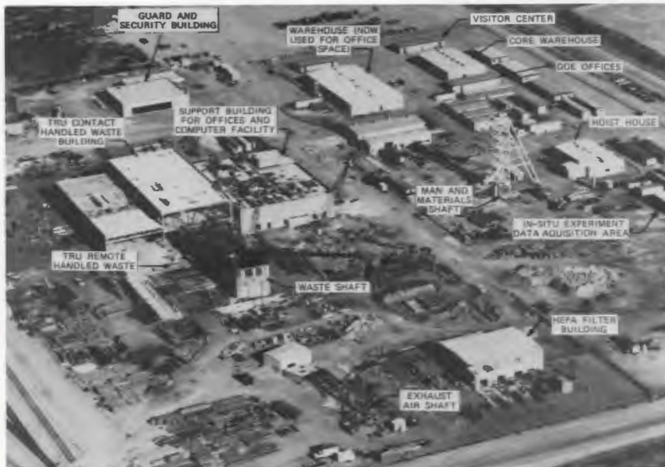
The Waste Isolation Pilot Plant (WIPP), a federal repository for transuranic (TRU) wastes, has been under construction since 1983 in Carlsbad, New Mexico. Beginning in the early 1990s, the facility will accept TRU wastes for permanent disposal. The wastes will be carried underground through the "waste shaft." Sources of these wastes are ORNL and other research, defense, and manufacturing facilities throughout the nation.
