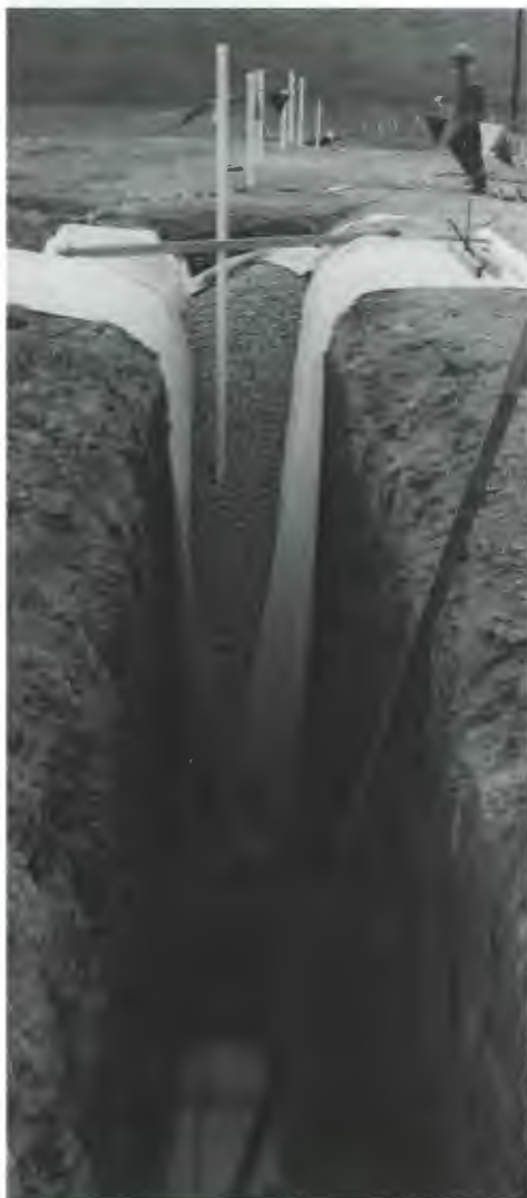
A view of the solid waste storage area (SWSA) No. 6 French drain during construction. The 1-m wide excavation is lined with filter fabric, backfilled with crushed stone, and covered to original grade with excavated soil. The drain was found to protect half of the burial site for low-level radioactive waste (and 29 of 49 trenches) from contact with rising groundwater.
