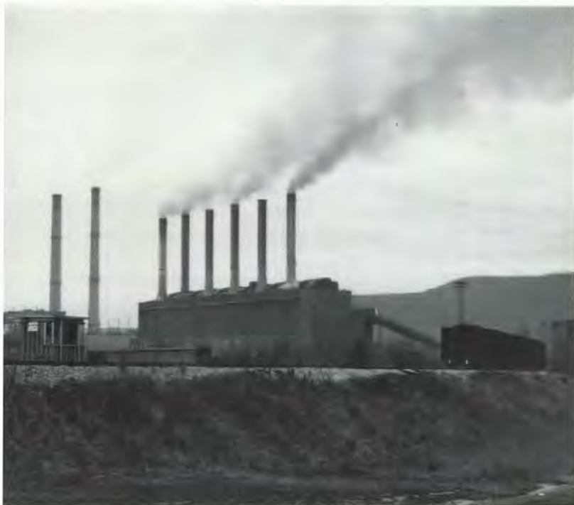
Coal-burning plant in the eastern United States spews sulfur dioxide and nitrogen oxides into the atmosphere. These gases are the main contributors of acidity in rainfall.
