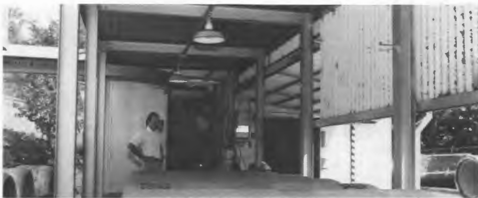
Dan Kearney (left) and Williams check the chlorine storage tanks at the pump station on the Clinch River. Water is chlorinated at the river near Clark Center Recreation Park before being pumped to the treatment plant on top of the hill, where more chlorine is added. Kearney is with the Construction Division of the Department of Energy's Oak Ridge Operations, and Williams is water plant superintendent with Rust Engineering Company.
