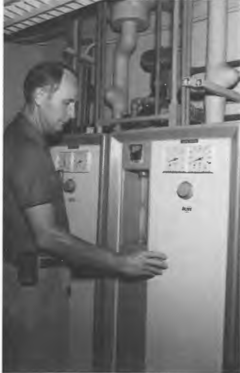
At Oak Ridge's water treatment plant, Hal Williams adjusts the rate of flow of chlorine into the drinking water. Above are "feeders," small pipes that add chlorine to the water as it enters the storage reservoir.
