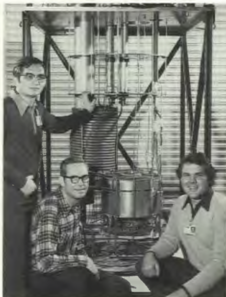
Winston Lue, Bob Brown, and John Miller, with their 8T experimental magnet wound with a cable-in-conduit conductor.
