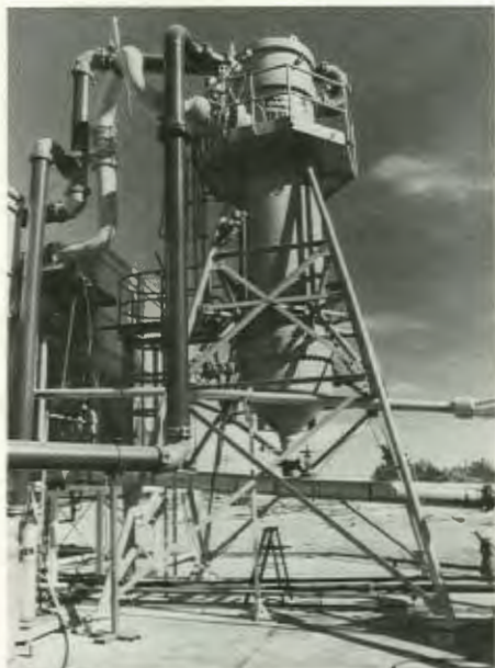
This loop at the East Mesa, California, geothermal test site was used to test fluted tubes designed at ORNL. These tubes were tested in a condenser ten times the size of the pilot-plant condenser at DOE's Raft River, Idaho, geothermal test site, where one of ORNL's high-performance tubes was first evaluated.
