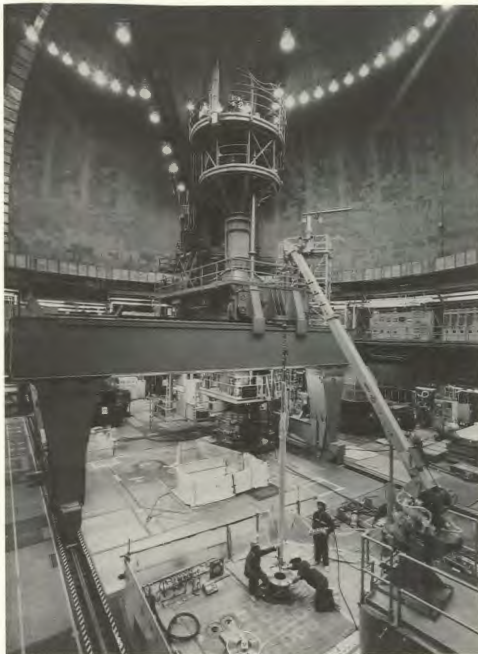
Inside the Fast Flux Test Facility in Richland, Washington, is a sodium-cooled reactor for testing fuels and materials under normal operating conditions. ORNL provided guidance in the design of the FFTF shield.
