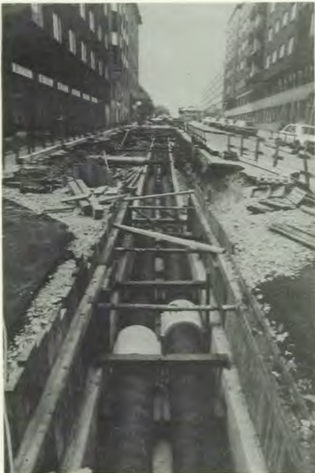
In Uppsala, Sweden, installation of district heating piping is an ongoing process.
