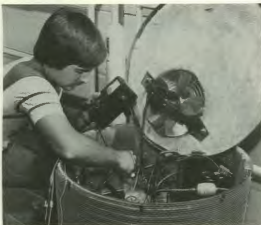
This heat pump-water heater being installed at ORNL's Energy Conservation Laboratory was developed by industry under ORNL's guidance and is now available commercially. It saves up to half of the energy used by a conventional resistance-type electric water heater.
