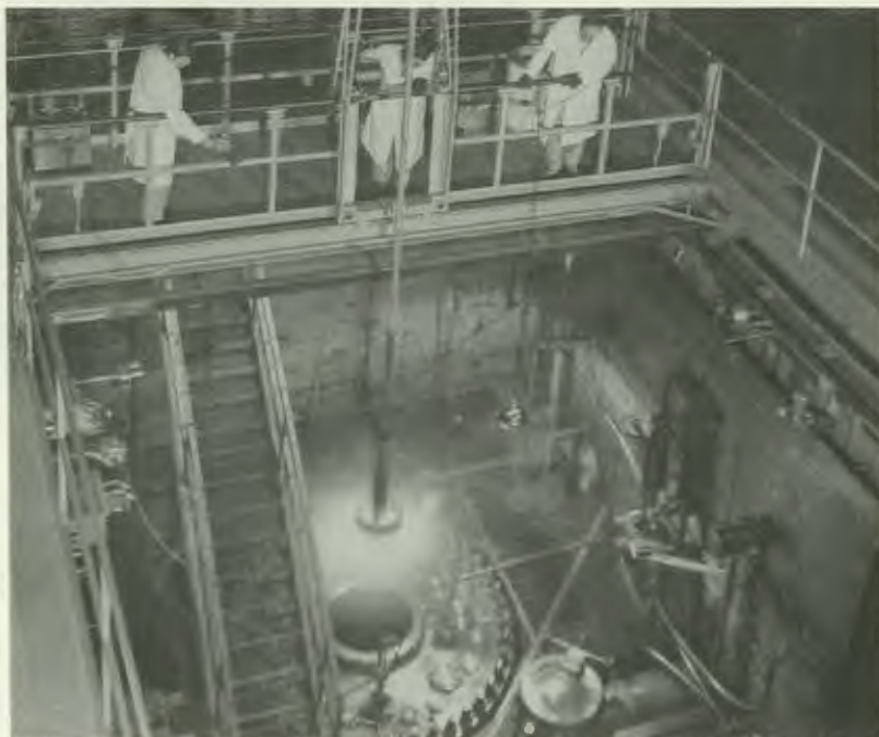
Reactor operators use a small crane to remove a fuel element from the High Flux Isotope Reactor.
