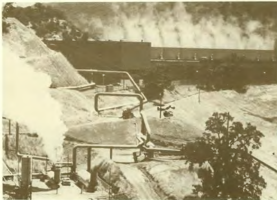
Vapor plumes and pipes dominate this view of the 100-MW geothermal power plant at Geysers, California, north of San Francisco. About 80% of the geothermal steam escapes to the atmosphere rather than being returned to the ground.
