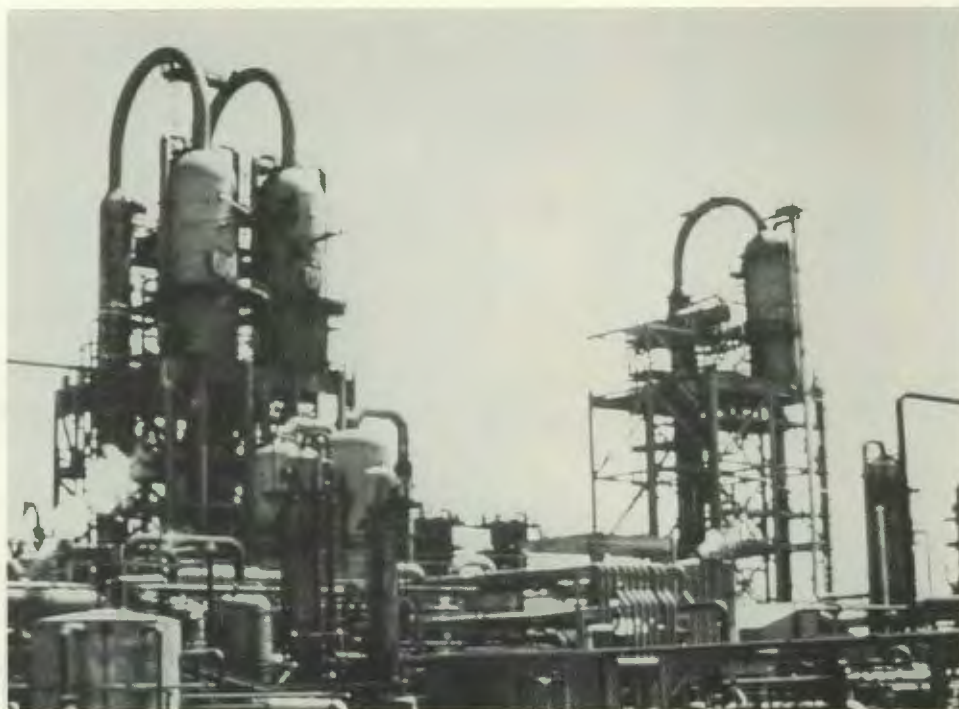
The Synthol synthesis reactors at SASOL with gas/oil absorption systems in foreground.
