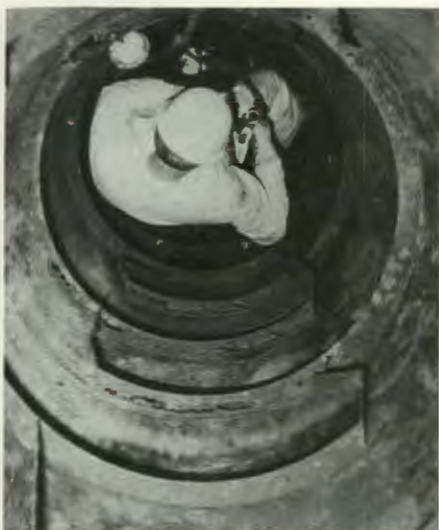
Maurice Allen inspects the corroded walls and tray supports of the wash solvent column at the Fort Lewis, Washington SRC-II plant.
