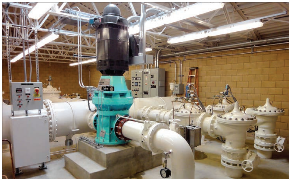
A hydropower turbine is installed into an existing drinking water distribution system in Palmdale, California. Image credit: Canyon Hydro
