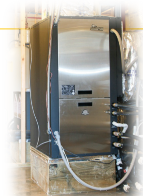
Prototype of ClimateMaster's Trilogy™ 40 Q-Mode™ while installed in ORNL research house
