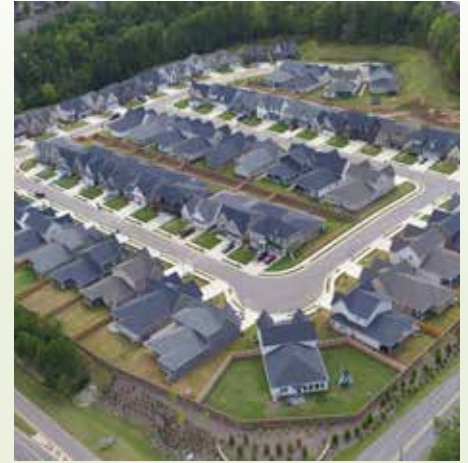
ORNL and Southern Company's Smart Neighborhood features a networked microgrid and transactive controls for intelligent load balancing.
