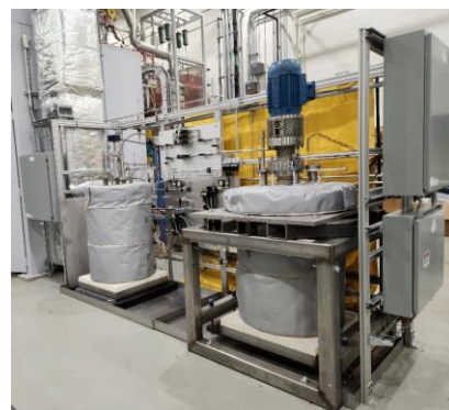
SPICEE with Bearing Test Rig Installed
