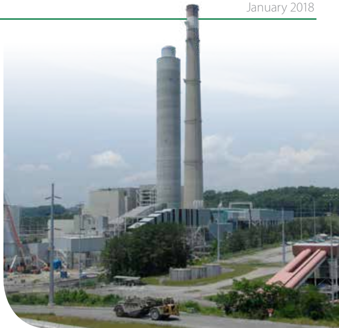
Tennessee Valley Authority's Bull Run Fossil Plant, a pulverized-coal supercritical power station in Clinton, Tennessee.
